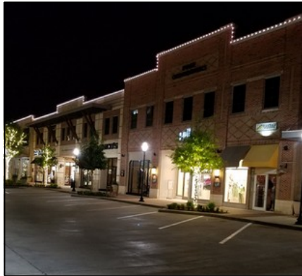
Downtown Lighting - Project 2.2
